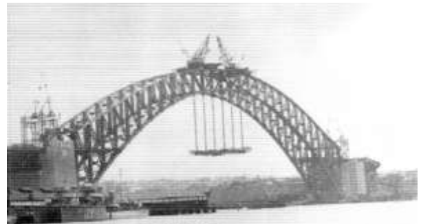
(d) Arch almost completed; gap being closed by easing out ropes one by one on both sides
